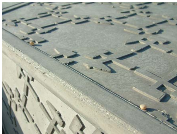
Photo 4: The Tettye-park furnishings' roughly chamfered edges
